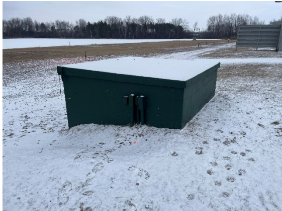
Figure 21 Side of Trap house with the Voice Plug.
