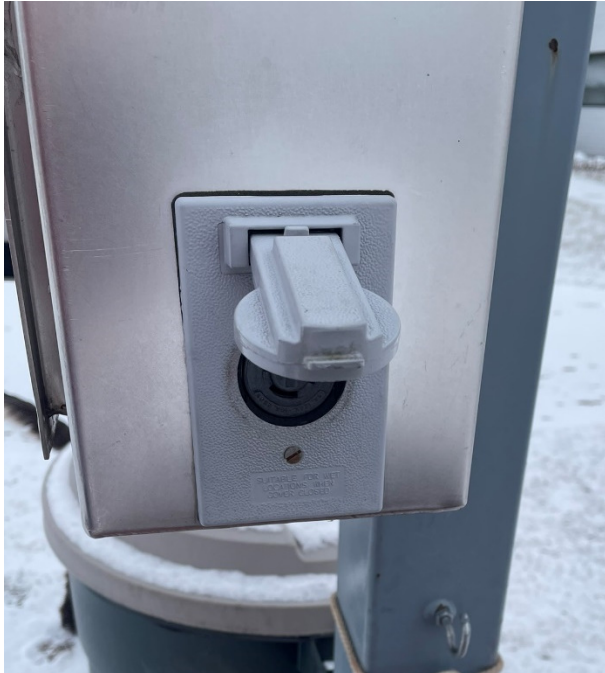
Figure 7 Skeet Plug and Strain Relief Hook
