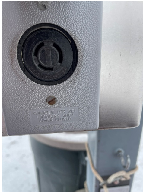
Figure 8 Twist Lock Skeet Plug Detail
