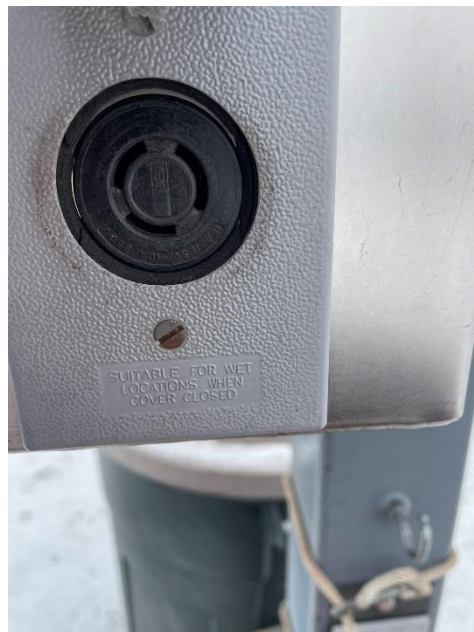
Figure 7 Skeet Plug and Strain Relief Hook
