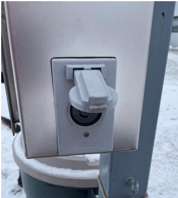
Figure 7 Skeet Plug and Strain Relief Hook
