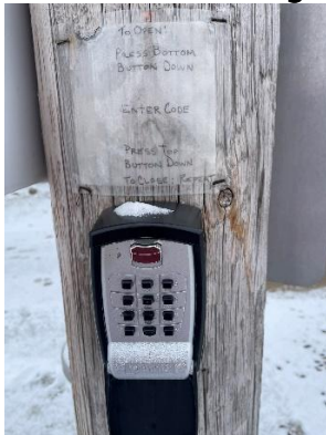
Figure 13 Lock Box to access the keys. Located on Light Posts 1, 3, 5, and 7
